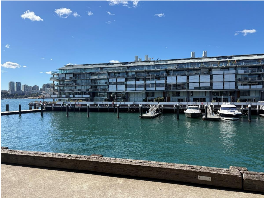
Figure 6: View of Pier 7 from east elevation of Pier 8
