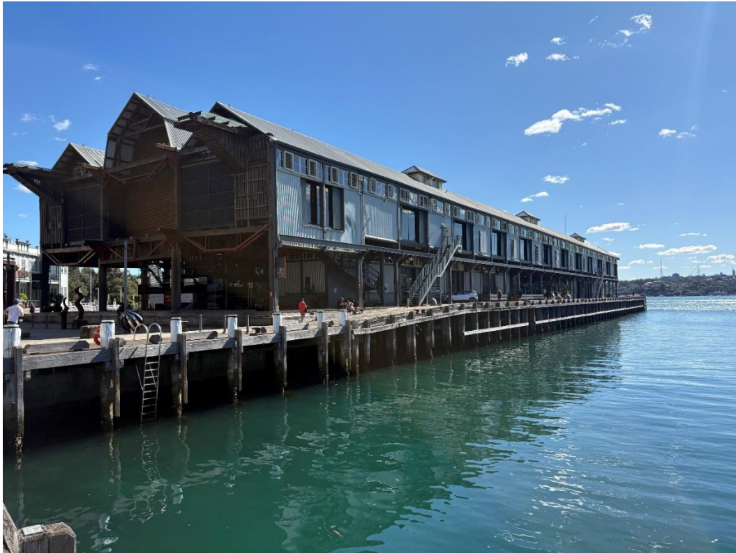
Figure 8: East elevation of Pier 8
